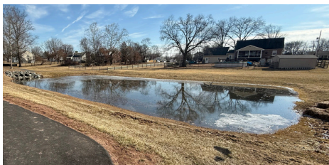
The basin pictured above was installed at Douglass Park in 2024 to help manage stormwater issues. Public Works is planning to convert this basin to a rain garden like the existing one at the park to further improve water filtration and recharge capacity utilizing trees, shrubs, and herbaceous plantings.
