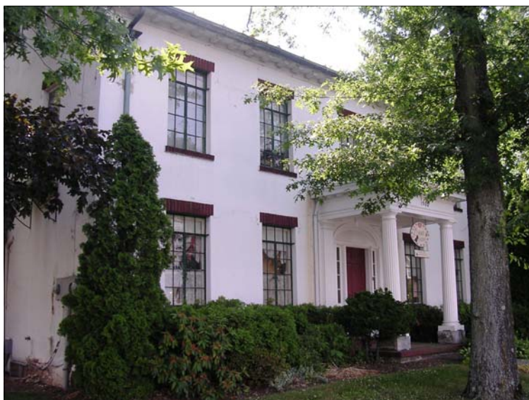
“The Corner Shoppe” at the intersection of Gilbertsville Road and E. Philadelphia Avenue gives the area a historic flavor.
